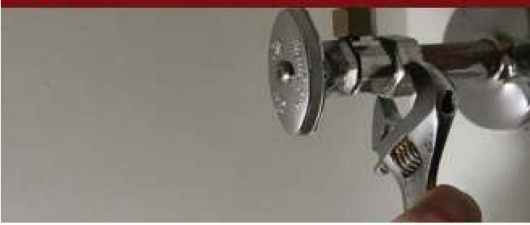
Figure 4: Install T's and Re-attach Angle Stops
