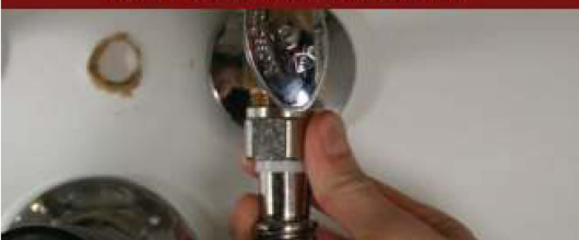
Figure 7: Install Flex Line to Flange
