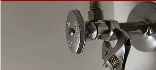
Figure 4: Install T's and Re-attach Angle Stops
