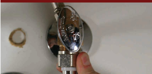
Figure 7: Install Flex Line to Flange
