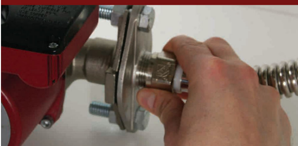
Figure 7: Install Flex Line to Flange
