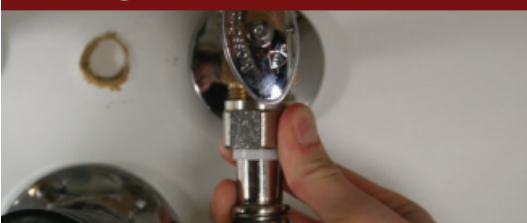
Figure 7: Install Flex Line to Flange
