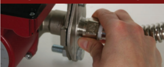
Figure 7: Install Flex Line to Flange
