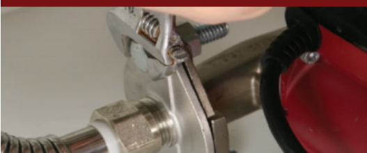
Figure 6: Install Flex Line to T
