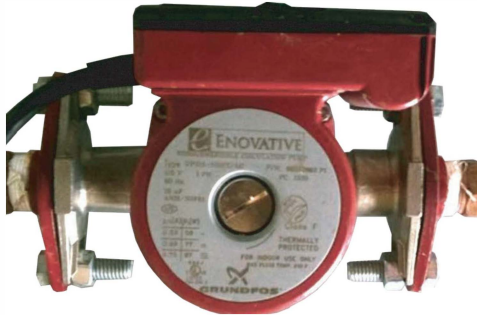
Figure 1: Pump on a return line
