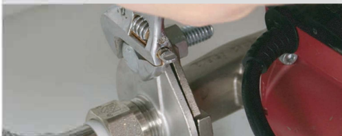
Figure 6: Install Flex Line to T
