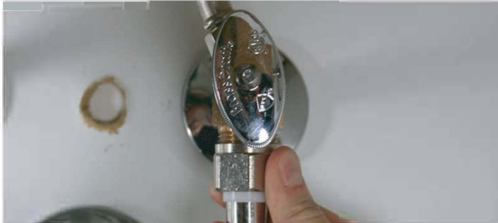
Figure 7: Install Flex Line to Flange
