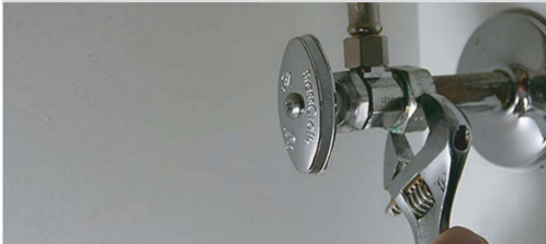
Figure 4: Install T's and Re-attach Angle Stops
