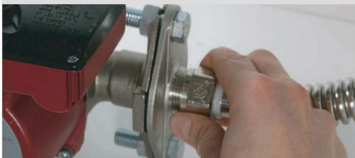
Figure 7: Install Flex Line to Flange
